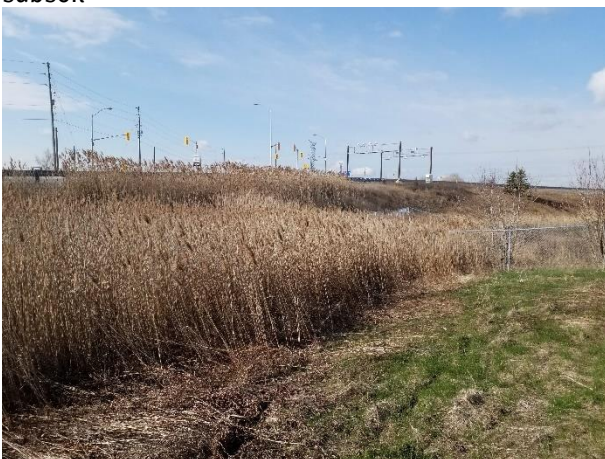
Plate 9: View across low and wet area with disturbed built up roadbed in distance.
